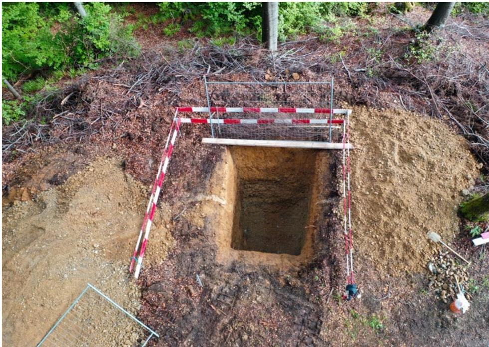
**Figure 3:** Photograph of the shallow trench at the Rütelbuck site. The depth of the trench is about 4.5 m.
